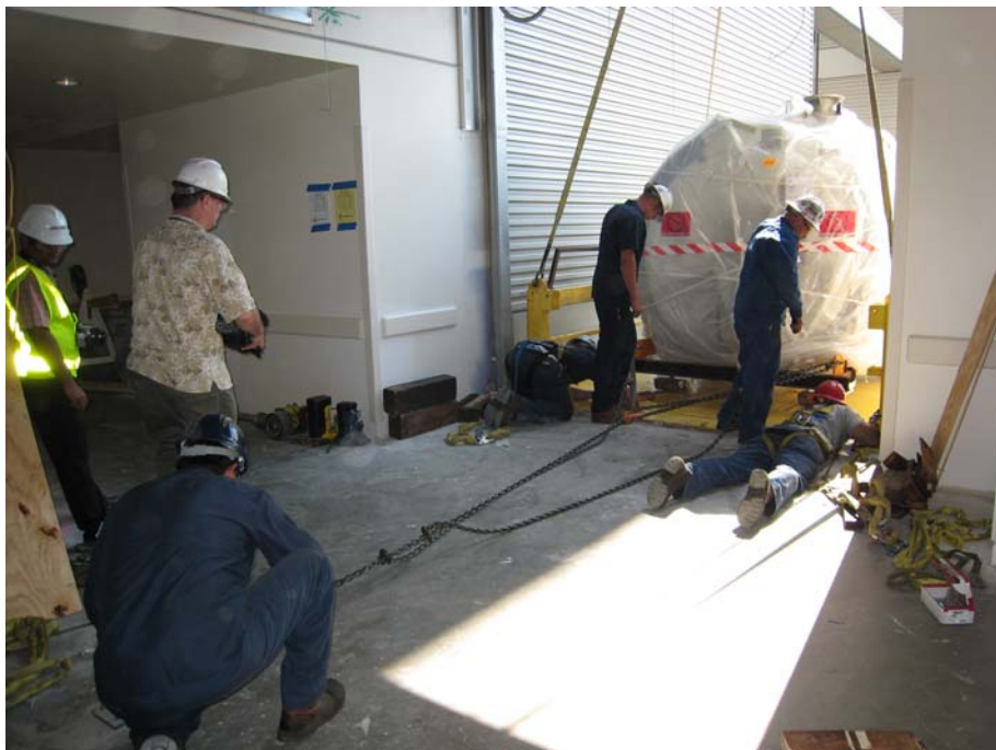
Using “Come-Along” to Retrieve MRI from Crane Pad
