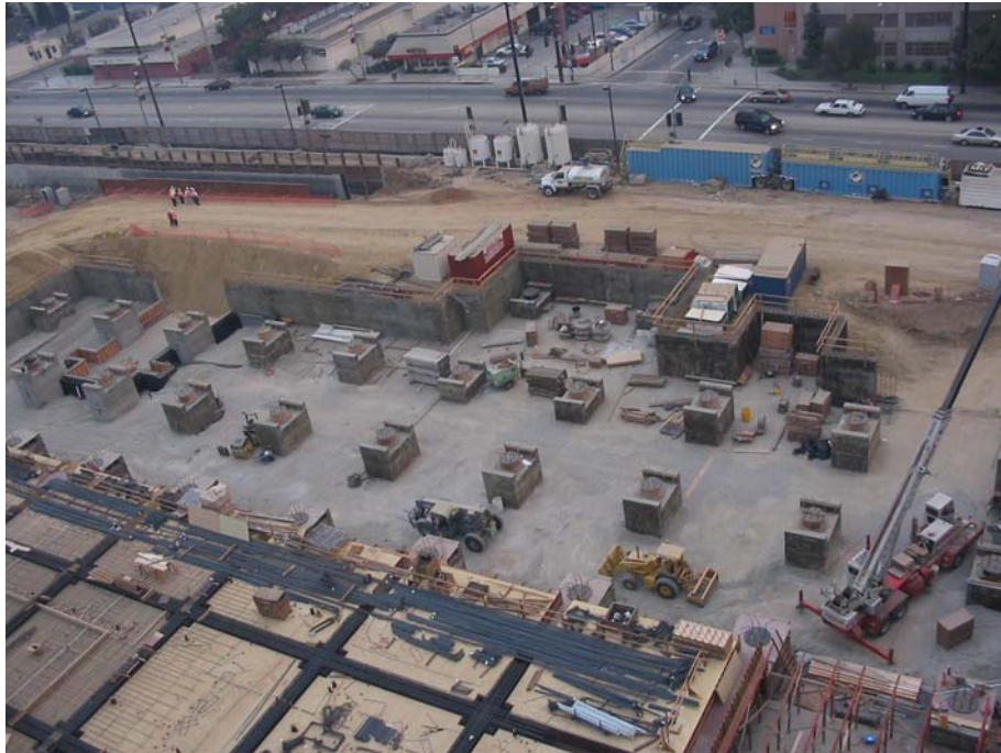
View of Base Isolators of Diagnostic & Treatment Building
