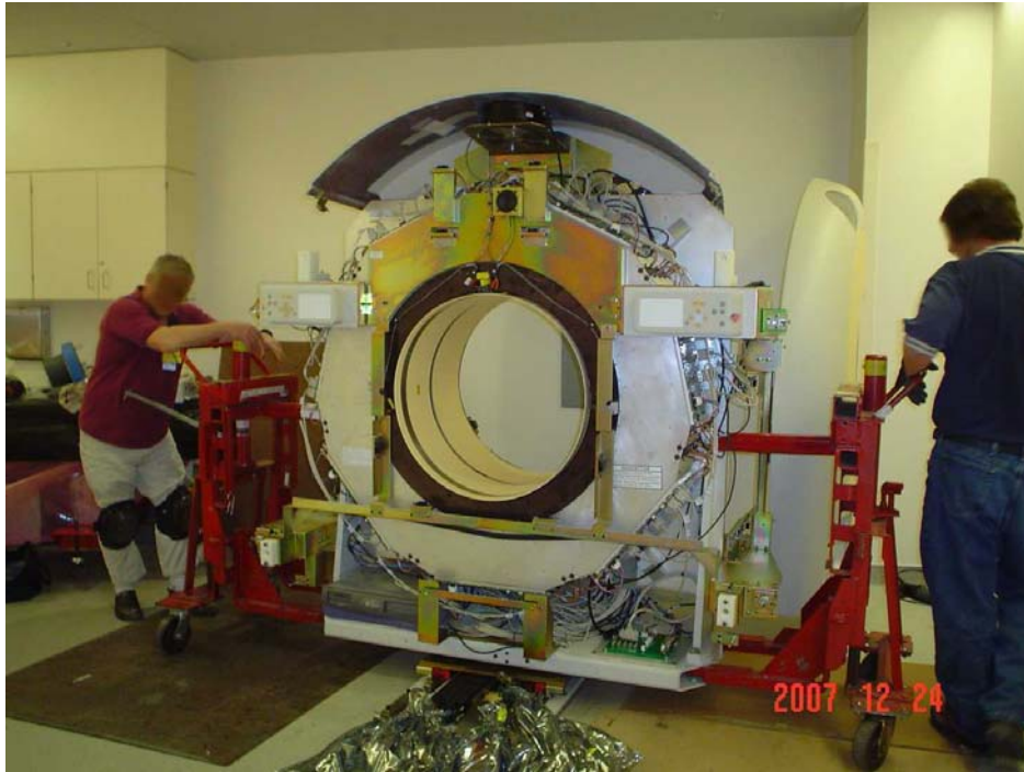
Phillips CT Scanner Installation
