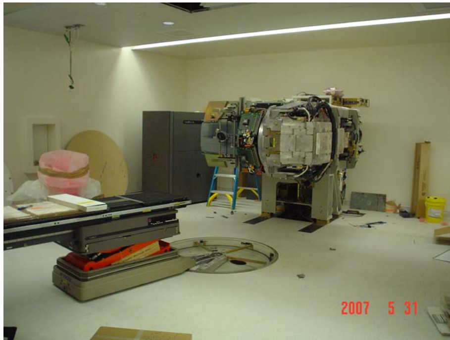
Linear Accelerator Installation in Progress
